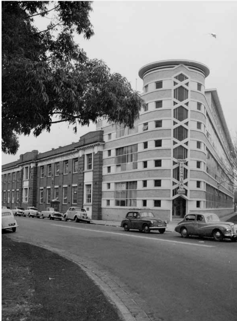
Caulfield Technical School E Block, architect Percy Everett, c.1950 (now Faculty of Art, Design & Architecture, Monash University)
